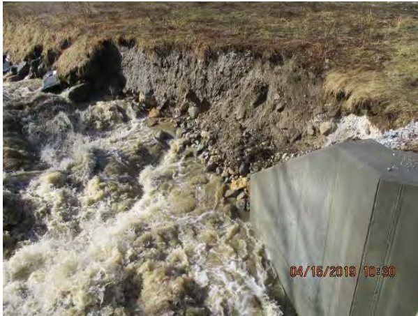
Bridge 25 Medway Road April 2019 Disaster
