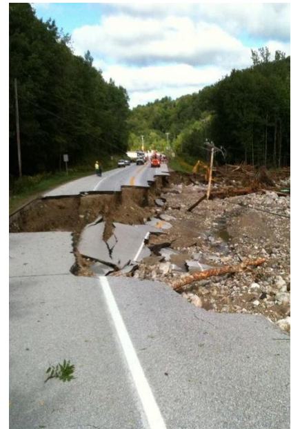
Image: Route 4 damage after Tropical Storm Irene.
