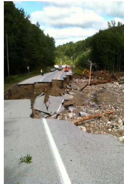
Image: Route 4 damage after Tropical Storm Irene.
