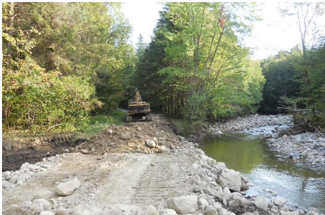
Image: Casella Construction rebuilding Wheelerville Road after Tropical Storm Irene.
