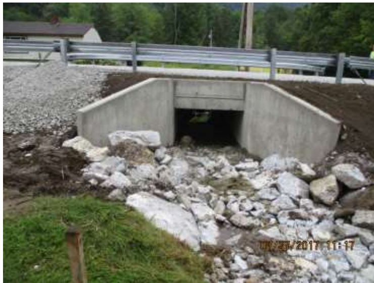
Culvert Replacement on Townline Road near Connor Drive
