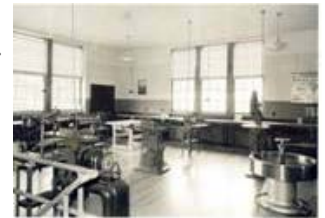
One of the vocational training rooms
